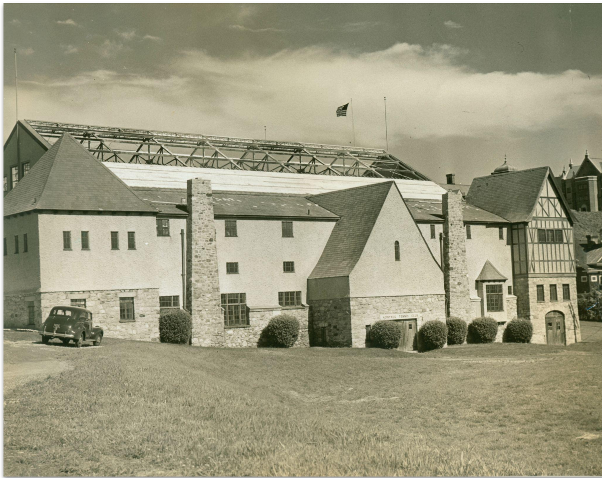
1940s roof repair
