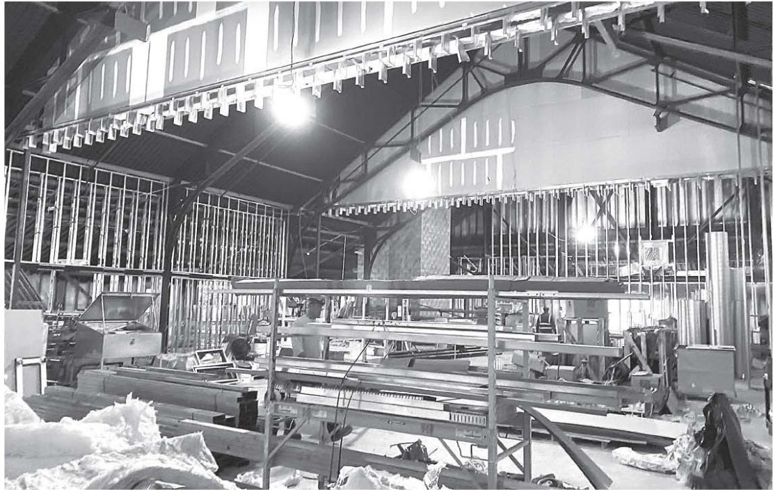
The Montauk Playhouse Community Center's second-floor cultural center is under construction.
