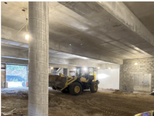
An excavator is at work on a lap pool on the lower level.
